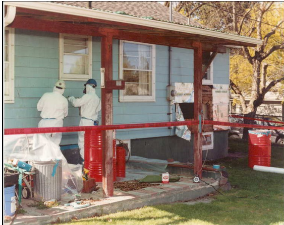
Prying to expose nail heads
