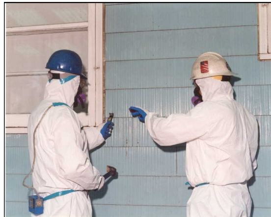
Pulling out nails
